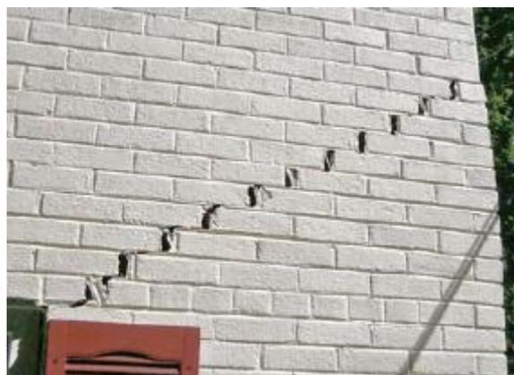
**Figure 1:** Foundation wall cracks
