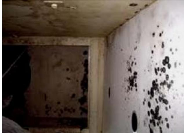
**Figure 9:** Fungi on internal wall
