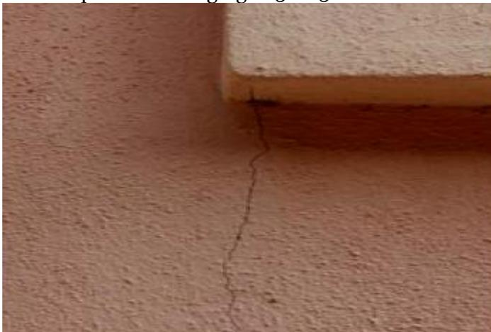
**Figure 3:** Crack between bay window corners
