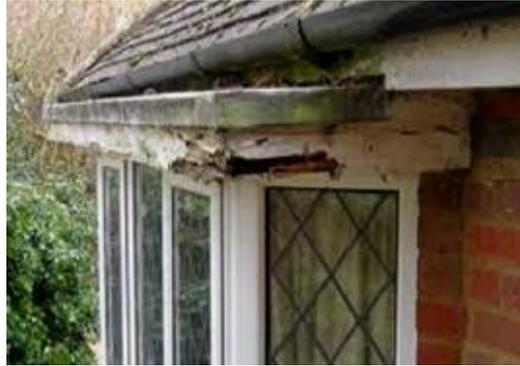
**Figure 7:** Timber decay of Flat roof
