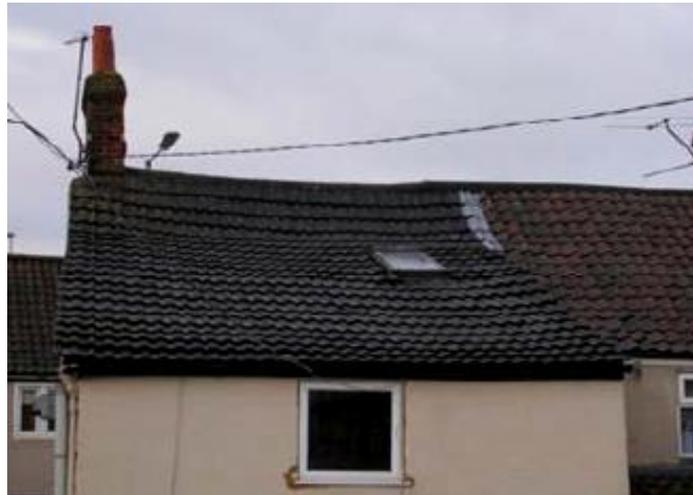
**Figure 10:** Sagging of roof
